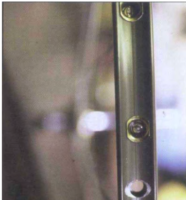
Countersinking the valve hole for tubulars
